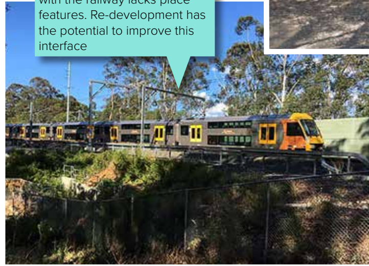
View towards the existing interface with the railway line.
