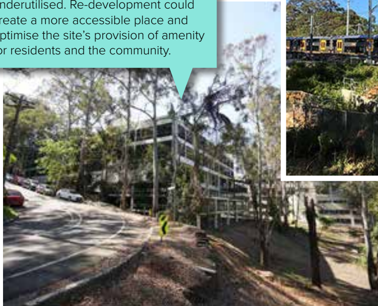
Looking north-east from Wongala Crescent towards underutilised part of the site.
